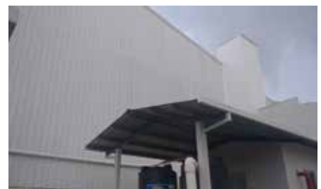
Rain Water Harvesting System at the Muthurajawela Warehouse
