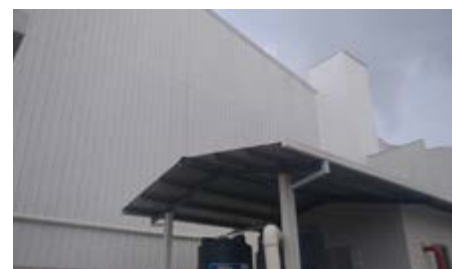
Rain Water Harvesting System
